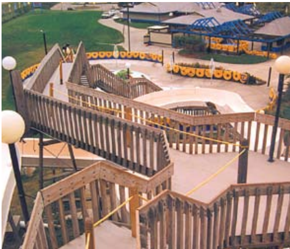
DURADEK® ON STEPS, WALKWAYS AND RAMPS OF WATERSLIDE PARK
